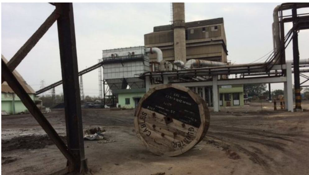
The plant is projected to save 60,000 tonnes of CO 2 emissions a year
